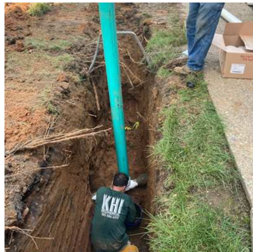
Installing one of the check valves.
