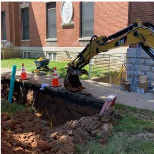
Plumbers dug the trench to access the underground pipes.
