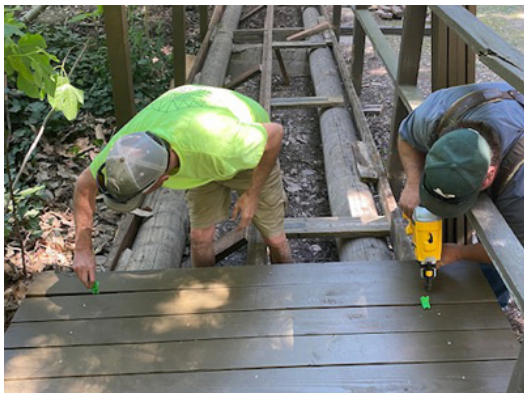
Volunteers work on replacing the boards of the bridge.
