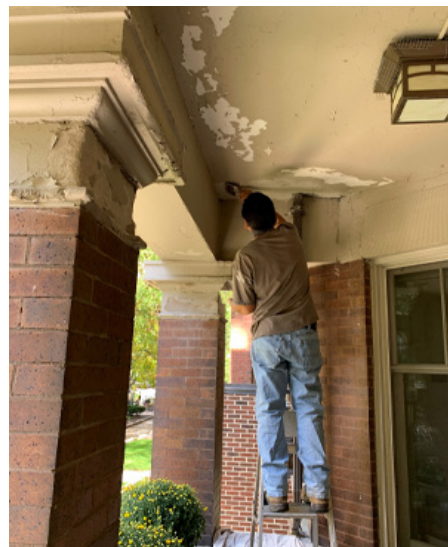
Crews scrape the loose paint from the ceiling of the porch to prepare for its weatherproofing.
