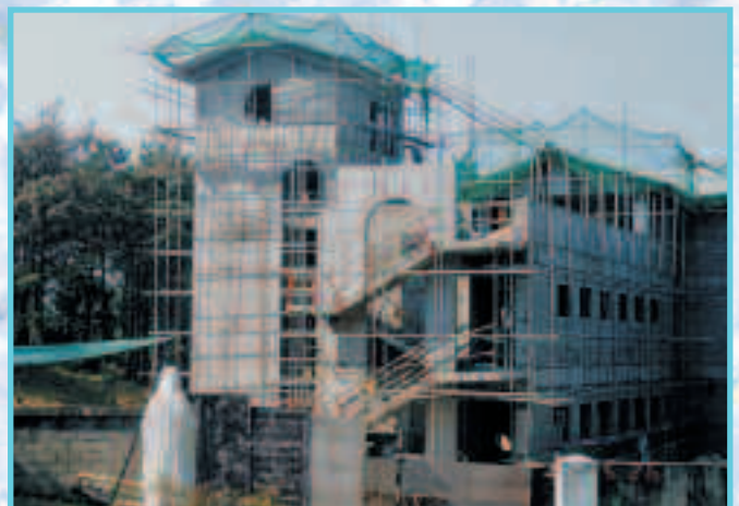
Construction of the monastery of the Passionist nuns in Korea
