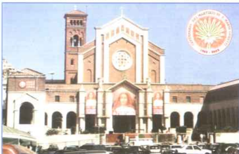
The Sanctuary of Nettuno
